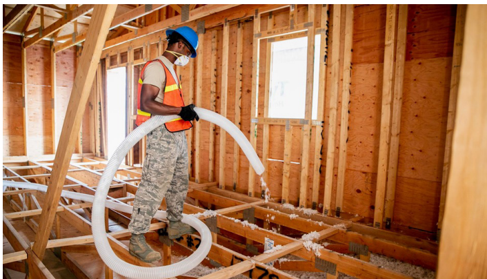
Innovative Readiness Training program crew member blowing insulation in the floor. Credit: Daniel Martinez
