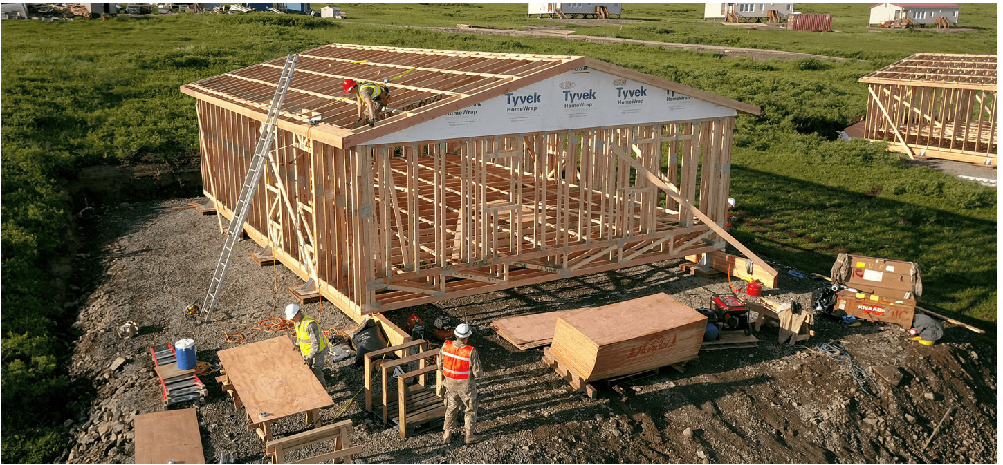
Framing of house by the Innovative Readiness Training program.
