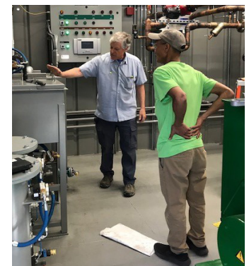
Xavier John speaking with an engineer in Mertarvik's power plant module.
